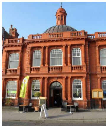
The Custom House, built in 1893, with terracotta ionic columns, balustrading and a copper dome.
